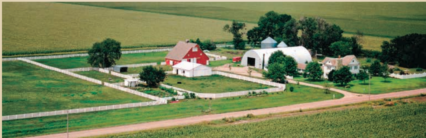
The original Country Estate Fence is the center section in this photo, installed more than 35 years ago.
